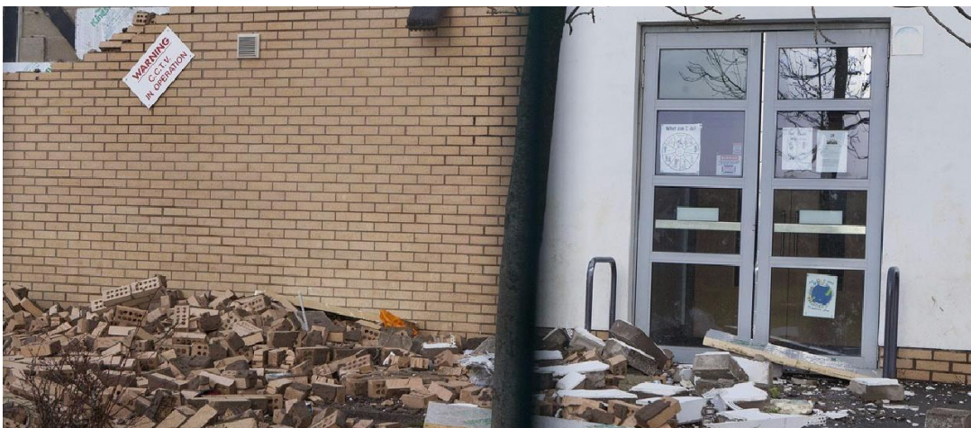
Image 4: Photograph taken at Oxgangs School of the gable wall after the collapse.
