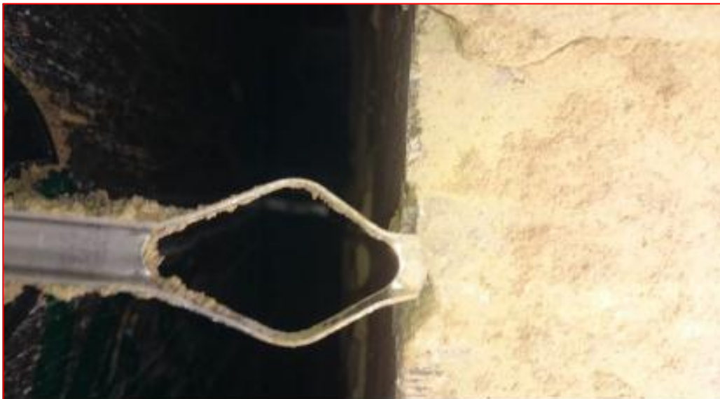
Photo 0185 Location 61A – Embedment 0mm
