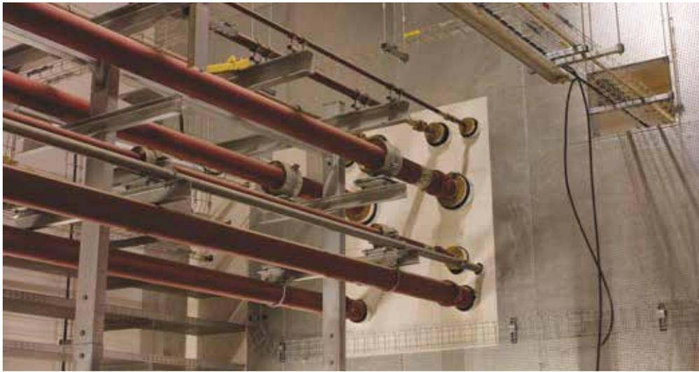
There are two types of fire protection, active and passive. Active fire protection typically suppresses a fire with sprinkler systems or, in some cases, by limiting the amount of oxygen in a space, whilst passive fire protection involves encasements, barriers and reactive coatings and products to hold back a fire, including any hot gasses and smoke.
