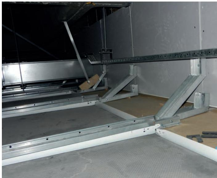
The manufacturer's recommendations have not been followed here and the metal ceiling has started to collapse.
