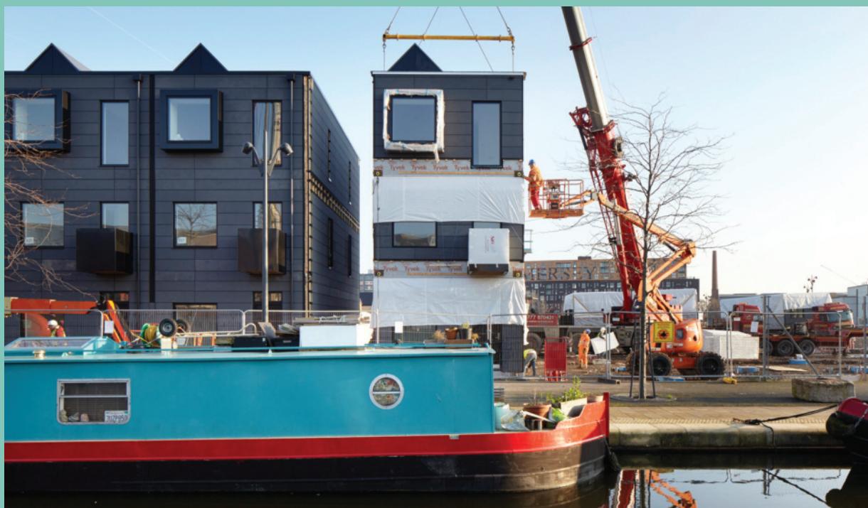
hoUSE, New Islington, Manchester
