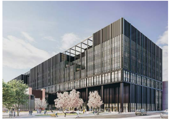
Figure 34 Manchester Engineering Campus development (MECD)
