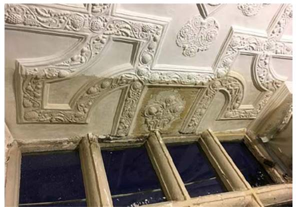
Figure 1: a traditional lath and lime Elizabethan ceiling during restoration.
