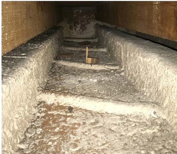
Figure 16: 1960s tray method with baton reinforcement.
