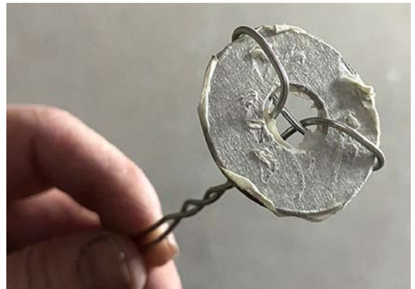
Figure 10: washer wire wrap method.
