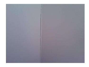
Other errors can occur when plaster is used in lieu of joint filler; the second coat of plaster can weaken the material in the joint causing cracks to appear later.
