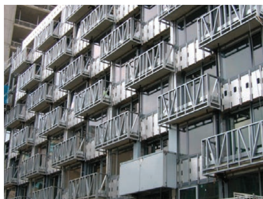
Figure 10.3 Light steel external walls with integrated balconies
