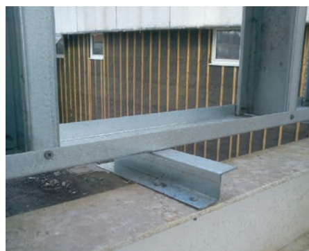
Figure 9.2 Z bar support brackets to infill walls along the line of the edge beam
