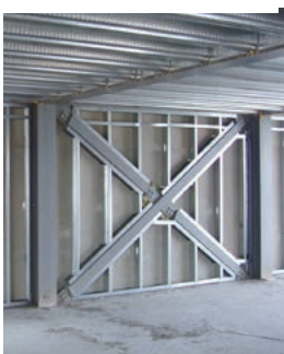
Figure 3.6 Infill walling around primary bracing
