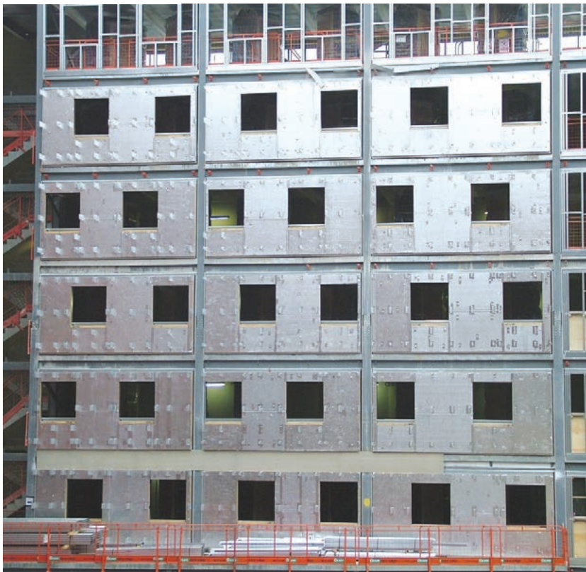
Figure 1.3 Typical prefabricated panelised external infill wall system
