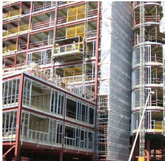
Figure 10.1 Curved infill walling - during and after construction
