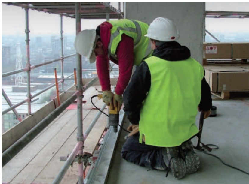
Figure 6.1 Fixing of base track to concrete slab
